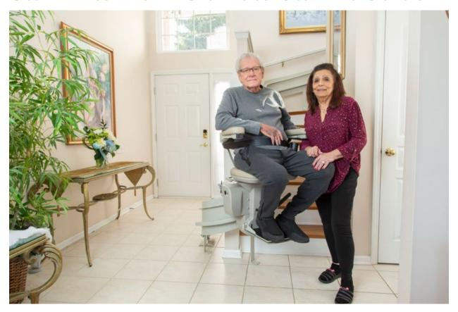
A <u>stair lift</u> is a battery powered, motorized chair that glides up and down a staircase on a rail mounted to the stair treads. Stair lifts can be installed indoors and outdoors in homes, churches, and other public buildings where permitted. Although, they are most popular for people with limited mobility that can no longer safely use the stairs at home. The typical user is able to stand, sit, and pivot with little to no assistance.
